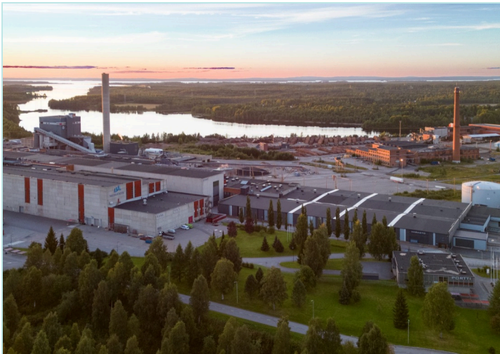
CSC office and data center in Renforsin Ranta Business Park, Kajaani. Photo: Mikael Kanerva, © CSC.
